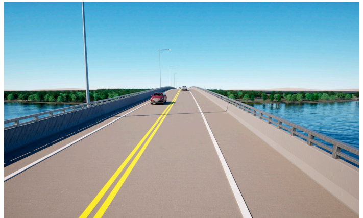
The new bridge will consist of one 12-foot wide travel lane in each direction with 8-foot wide shoulders.
