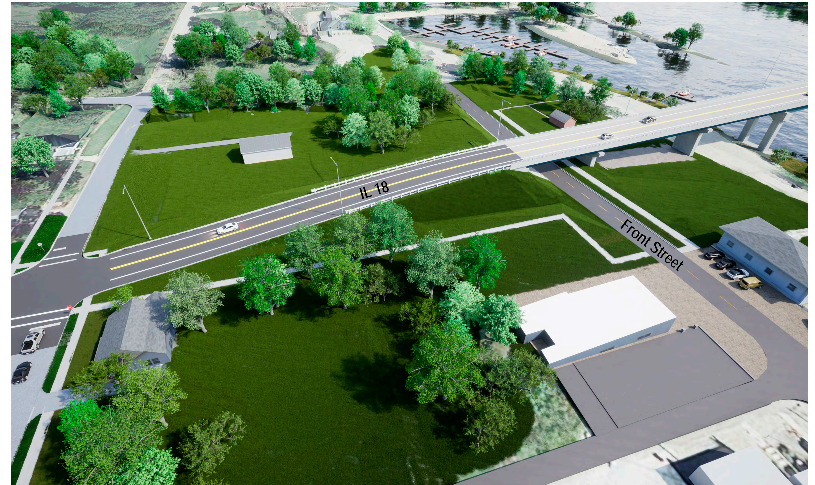
The new bridge will span Cromwell Drive and Front Street.
